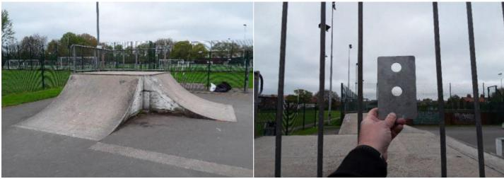
Finding: The horizontal opening in the barrier is in excess of Action: Repair the barrier 89mm and fails the requirements of BS EN 14974
