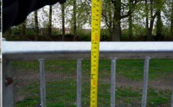
**Finding:** The height of the barrier is less than 1200mm and **Action:** Monitor - No remedial work recommended fails the requirements of BS EN 14974
