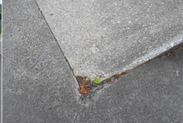
Finding: The riding surface of the ramp has some damage Action: Repair the affected areas apparent
