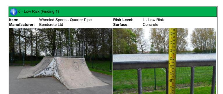
**Finding:** The height of the barrier is less than 1200mm and **Action:** Monitor - No remedial work recommended fails the requirements of BS EN 14974
