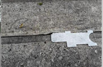
**Finding:** Joints between the riding surfaces should not be **Action:** Take corrective action to ensure that the gaps greater than 5mm to meet the requirements of BS EN 14974 between the joints do not exceed 5mm
