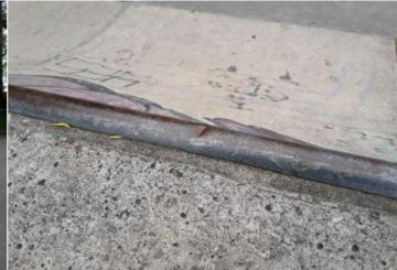
**Finding:** The coping has been damaged **Action:** Monitor for any further deterioration and replace as required
